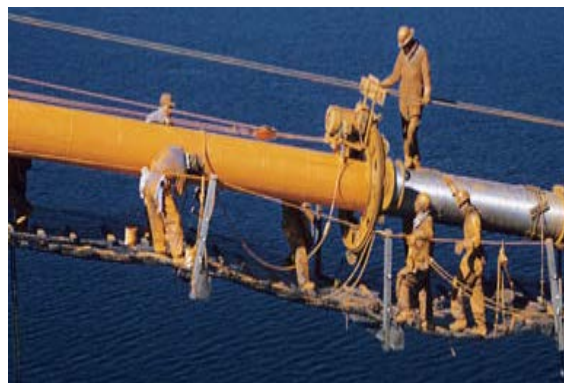
The bridge workers are coating it with paint
